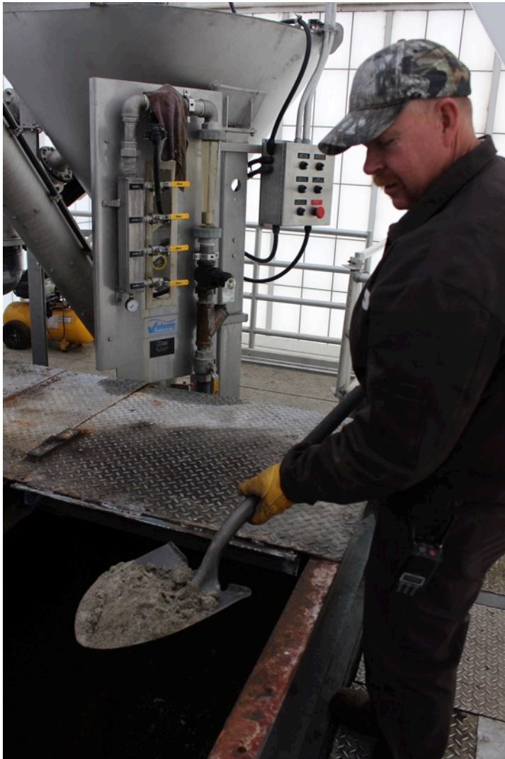
Lonnie Tucker, WPC plant operator, checks some of the screened material at the plant. The plant staff recently received two awards at a state conference.
