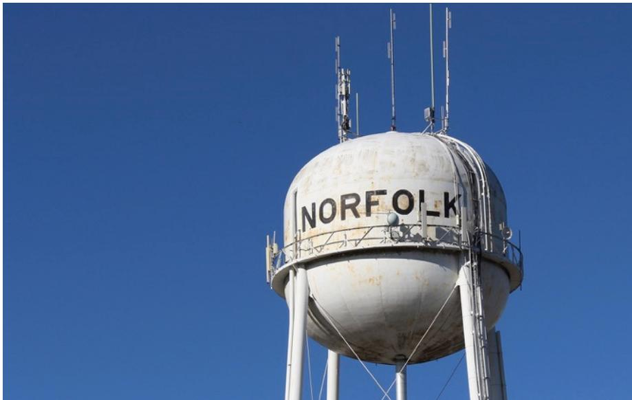
“Right now its main use is as a fixture to attach antennas onto. A galvanized antenna tower doesn’t have the upkeep as this tower and won’t need to be repainted in another 15 years like this one will need to be,” Watts said.
