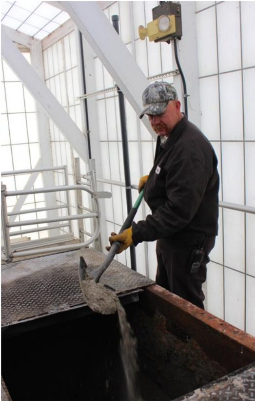
Lonnie Tucker, Water Pollution Control Plant Supervisor, shows the cleaned sand that was filtered out of the wastewater going through the plant.
