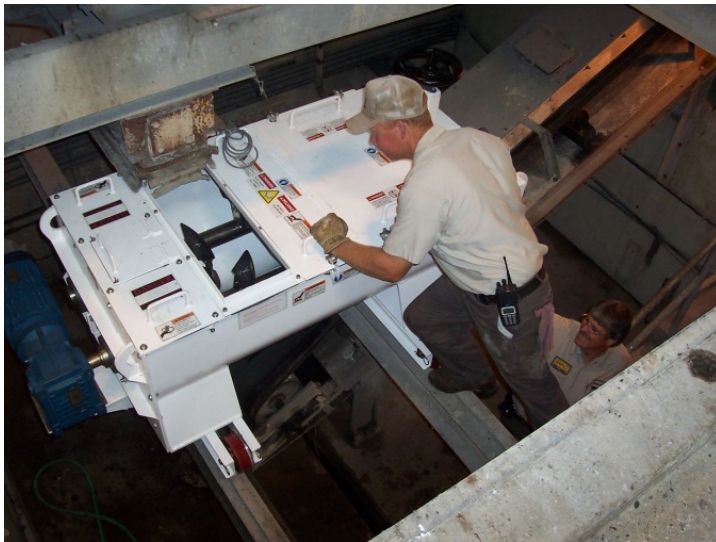
WPC Staff installing new blender
