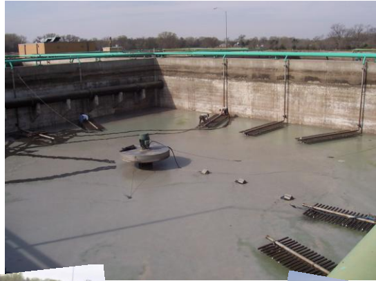
WPC Staff replacing diffusers in #2 SBR.
